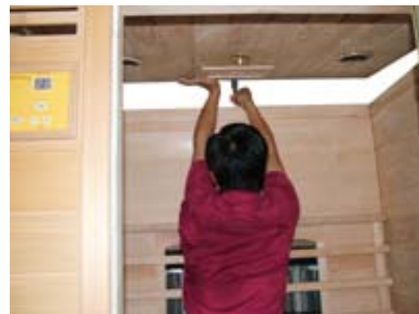
FIG-14 Leading the wires of heaters onto the board through the corresponding hole
