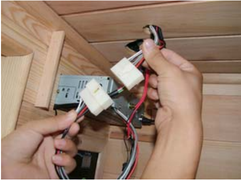
FIG-18 Link the CD connectors
