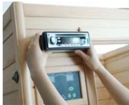
FIG-17.1 Fixing stereo w/ CD
