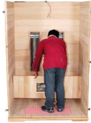
FIG-8 Assembling sitting board's support
