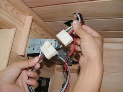
FIG-18 Link the CD connectors
